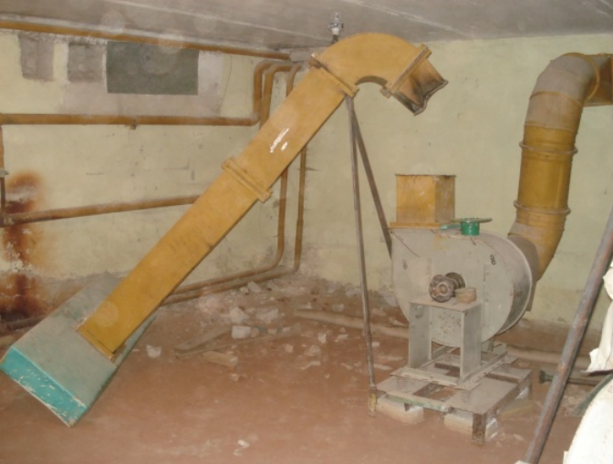
Ventilator exhaust
